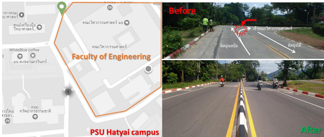
Figure 35 Example of road safety improvement in Songkhla: Case 2
